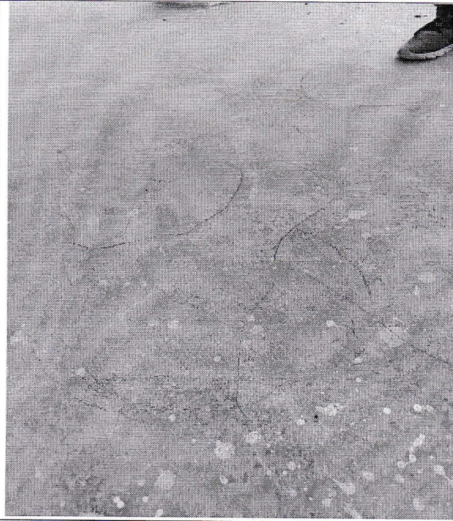
Cracks Appear in Corridor Floor
